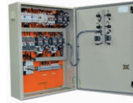
MOTOR CONTROL PANEL
